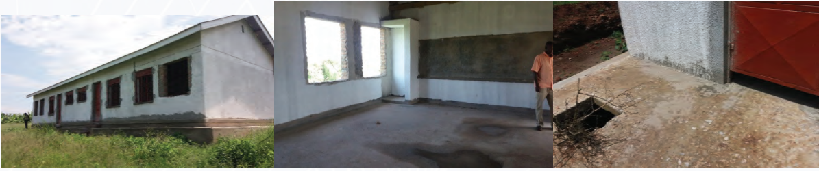
Source: IG; Construction of Primary School in Uganda in November 2020
