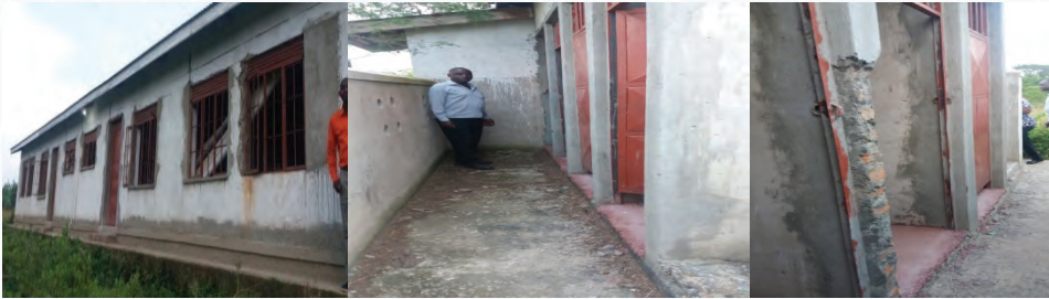
Source: IG; Status of construction of the Primary School in February 2022
